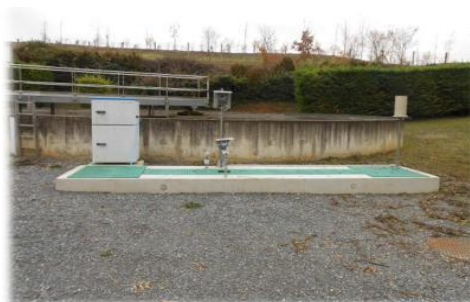
Figure 2. CANAL SORTIE DE STATION D'EPURATION
