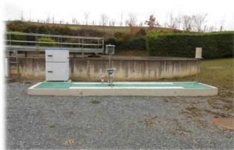
Figure 2. CANAL SORTIE DE STATION D'EPURATION
