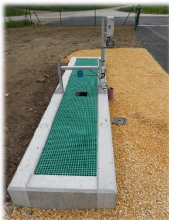
Figure 1. CANAL SORTIE DE STATION D'EPURATION
